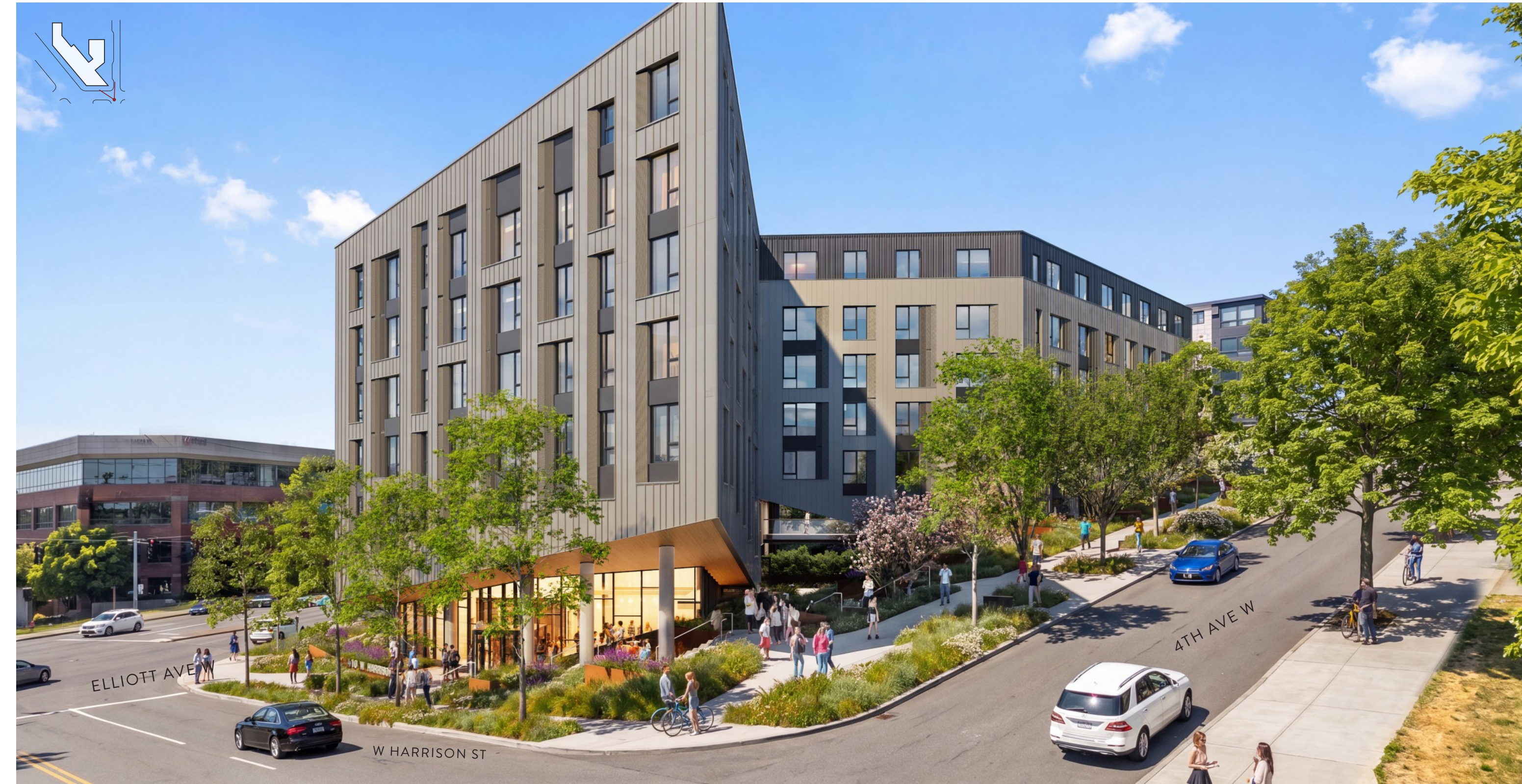
PROPOSED | Looking north at lobby on Harrison St and 4th Ave W
