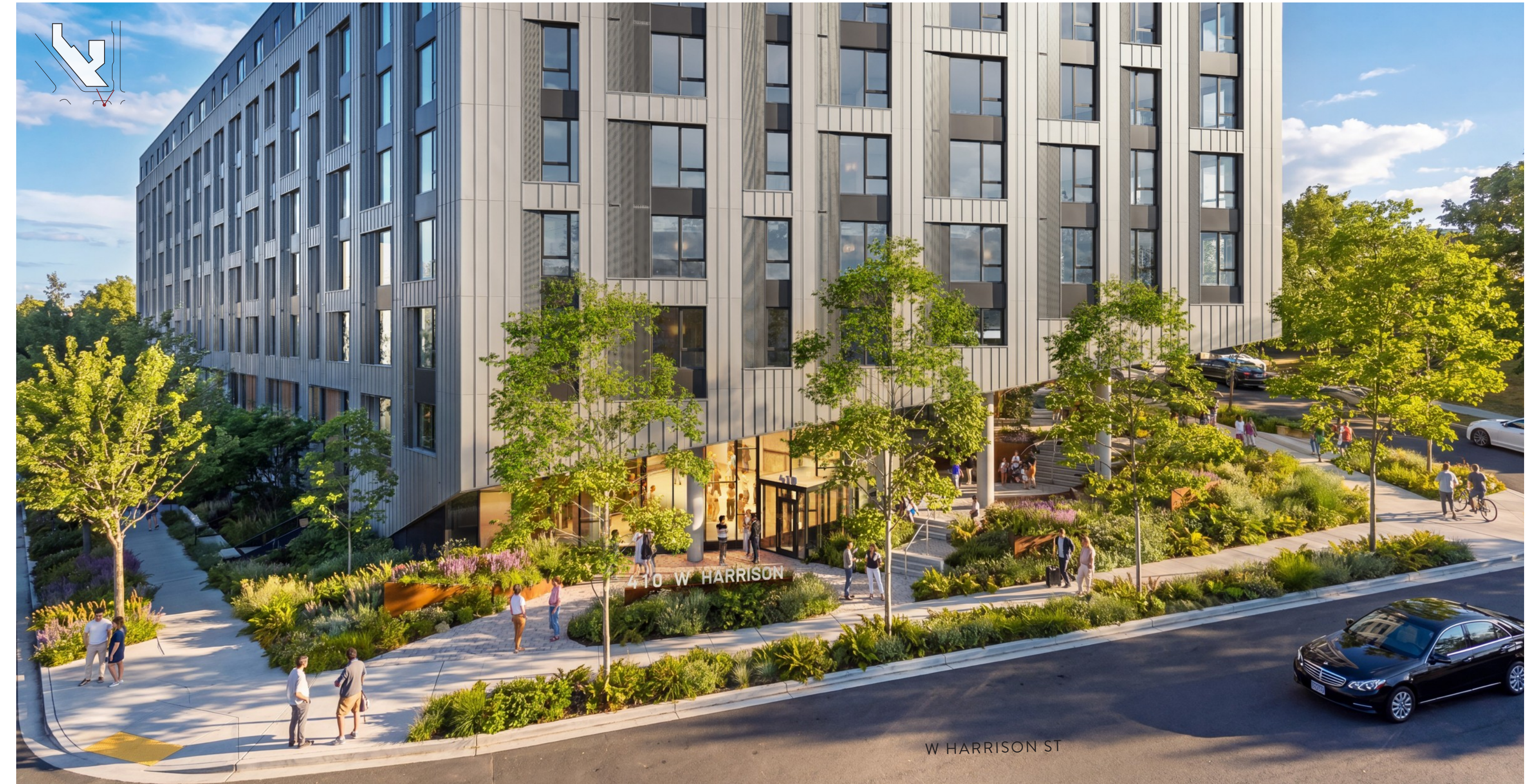
PROPOSED streetscape along Harrison St looking north, showing the pathway for pedestrians to "cut the corner" through the on-site landscaping.
