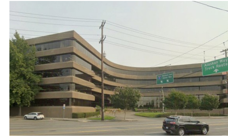
(E) * 300 Elliott Ave W (Office)
