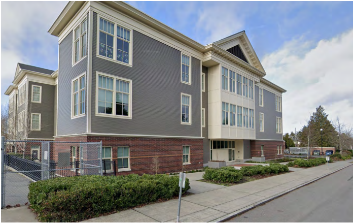
COE ELEMENTARY - CORNICE TRIM - USE OF BRICK AS BASE
