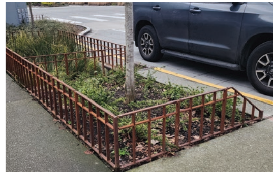
3. Planter Protection Railing
