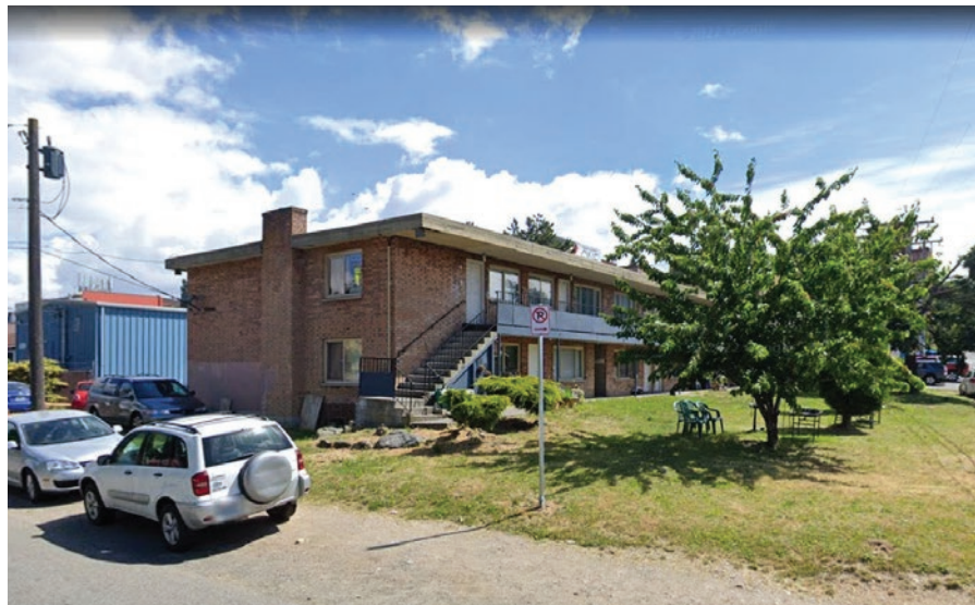
4. Naturally-occurring affordable housing on 32 Ave NE
