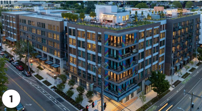
1 Tapestry Apartments 7 Stories Materials used: Red brick, gray and white metal panels, wood siding
