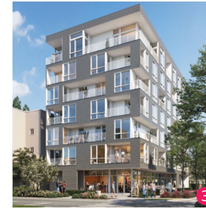
1100 NW 54th St- mixed use// under construction
