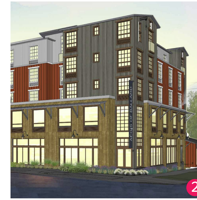
Aegis of Ballard- Senior Living // under construction
