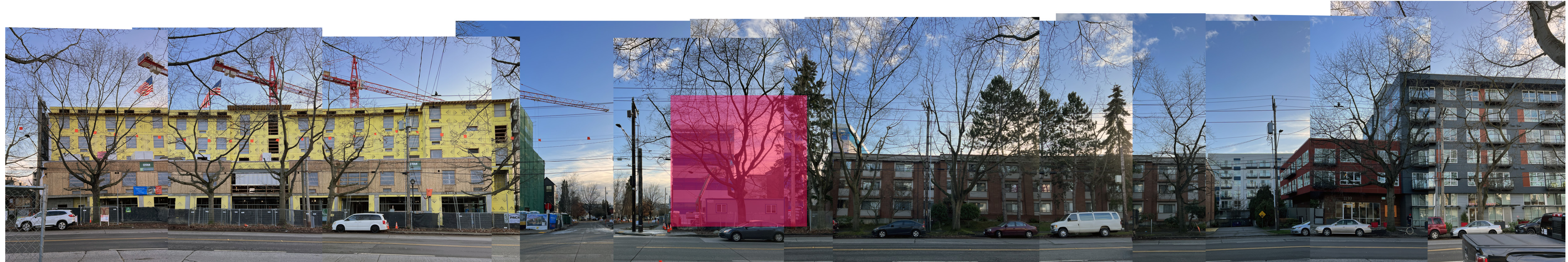
5-story multifamily building, under construction, Aegis senior living
