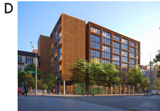
1722 BELLEVUE AVE IN PROGRESS
