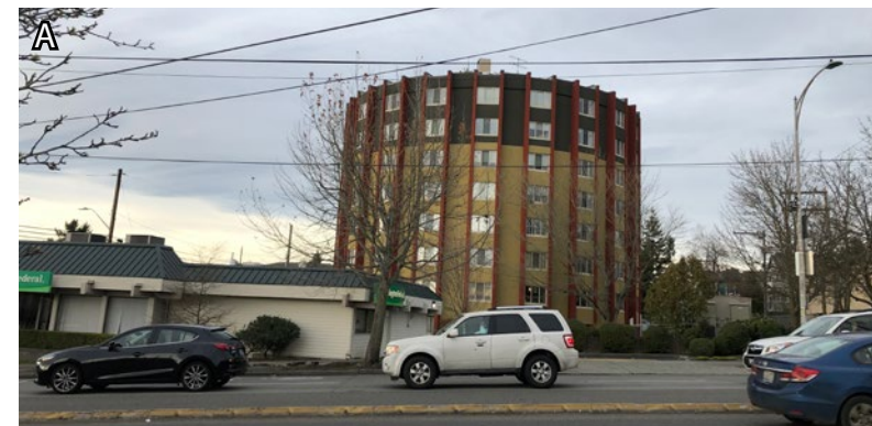
Cal-Mor-Circle An eight story, 75 unit apartment building that features affordable housing through Seattle Housing Authority.
