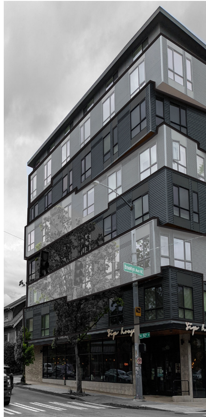
The Stax (5001 Brooklyn Ave NE) - shifting floor plate massing to create a more dynamic horizontal expression
