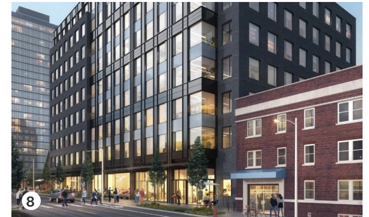
8 CHAPTER BUILDING II - 4536 BROOKLYN AVE NE
