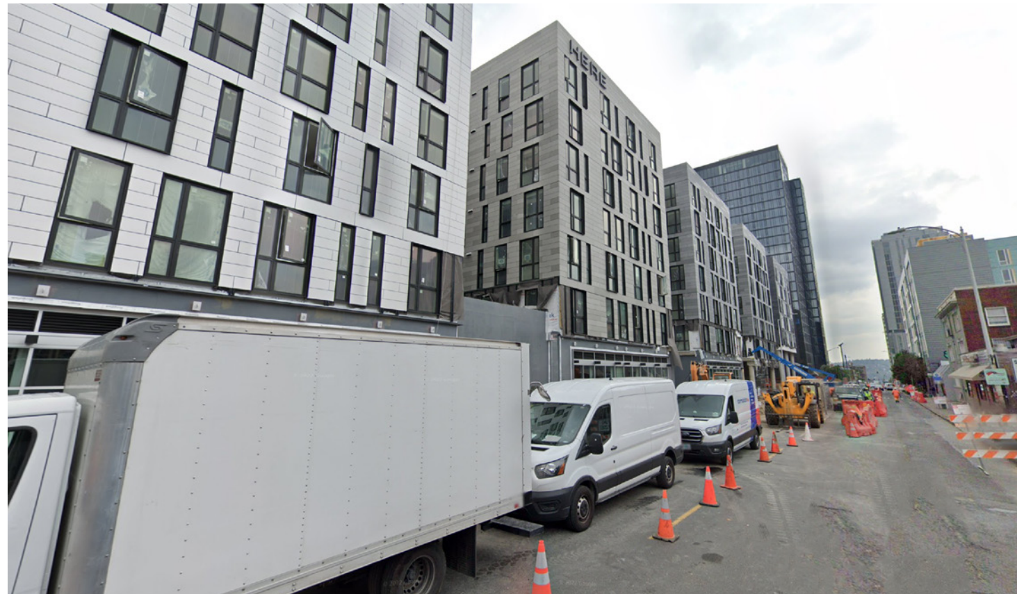
New multifamily mid-rise under construction mixed with older development in this transitioning neighborhood.
