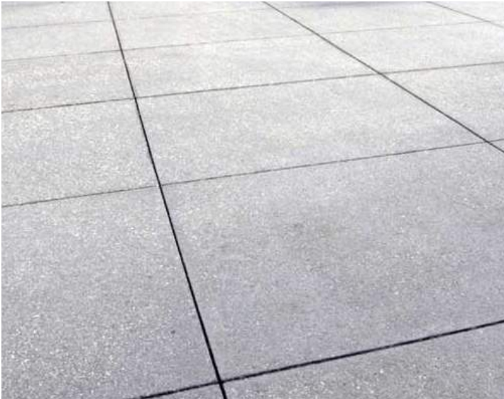
Saw-Cut Concrete
