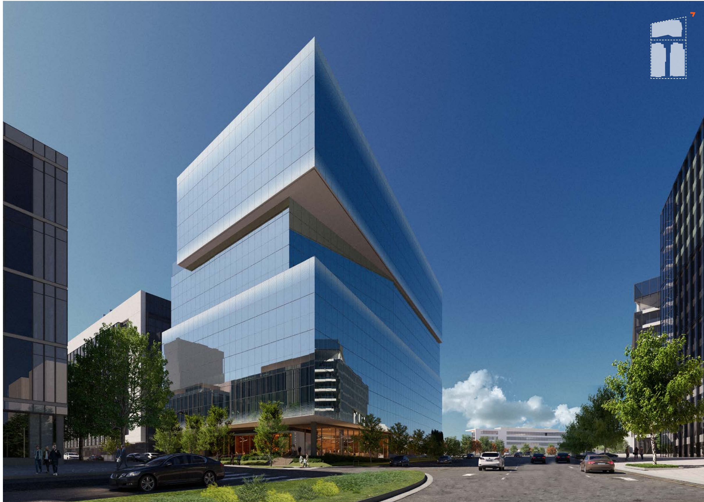
View of northeast corner from Mercer Street
