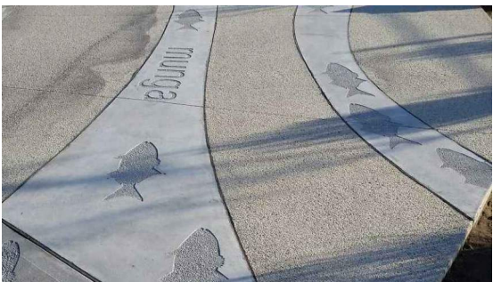
SANDBLAST IMAGES IN CONCRETE PLANTER WALLS AND PAVING
