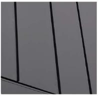
(2) FIBER CEMENT PANEL W/ METAL T FLASHING TRIM SW 7674 - PEPPERCORN
