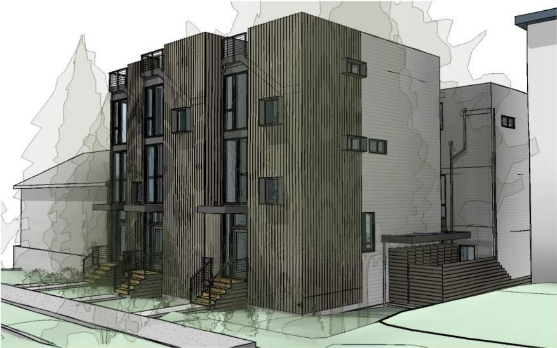
Greenwood Ave N units are staggered and wrapped with a rainscreen façade to reduce visual impact.
