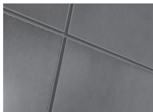
SMOOTH PANEL/ INFILL FIBER CEMENT PANEL COLOR: SW 7069 REVEALS BETWEEN PANELS: SW7069
