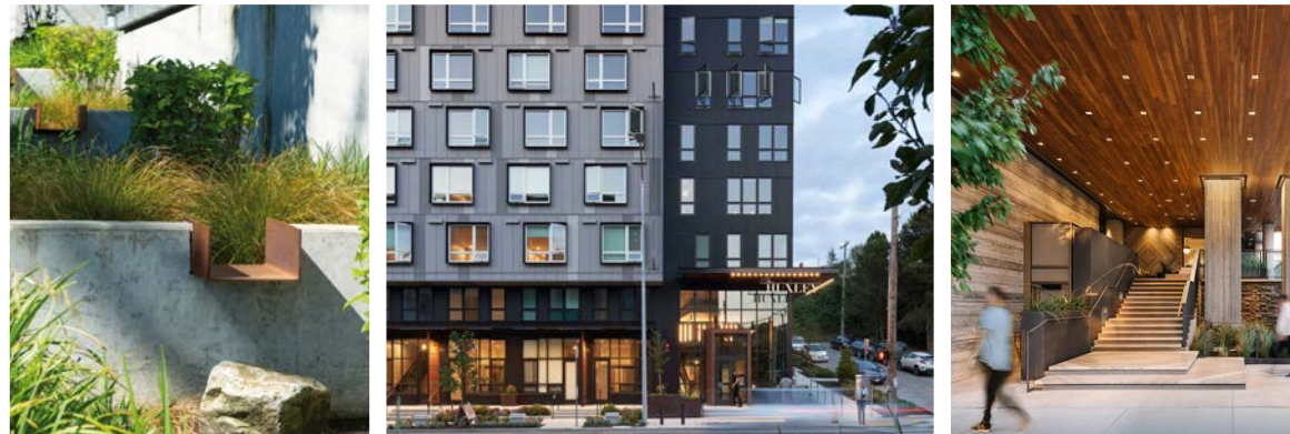
Artful drainage solutions and eroded corner mass celebrate the entry and provide visual interest that encourage sitting and watching the street.
