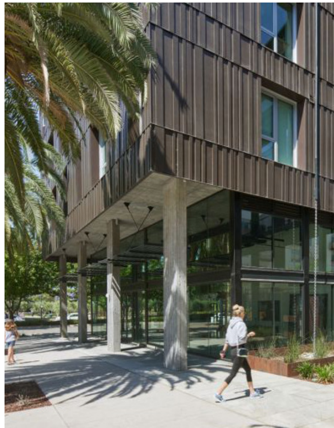
Recess lower level to provide weather protection and greater depth at sidewalk level for public life
