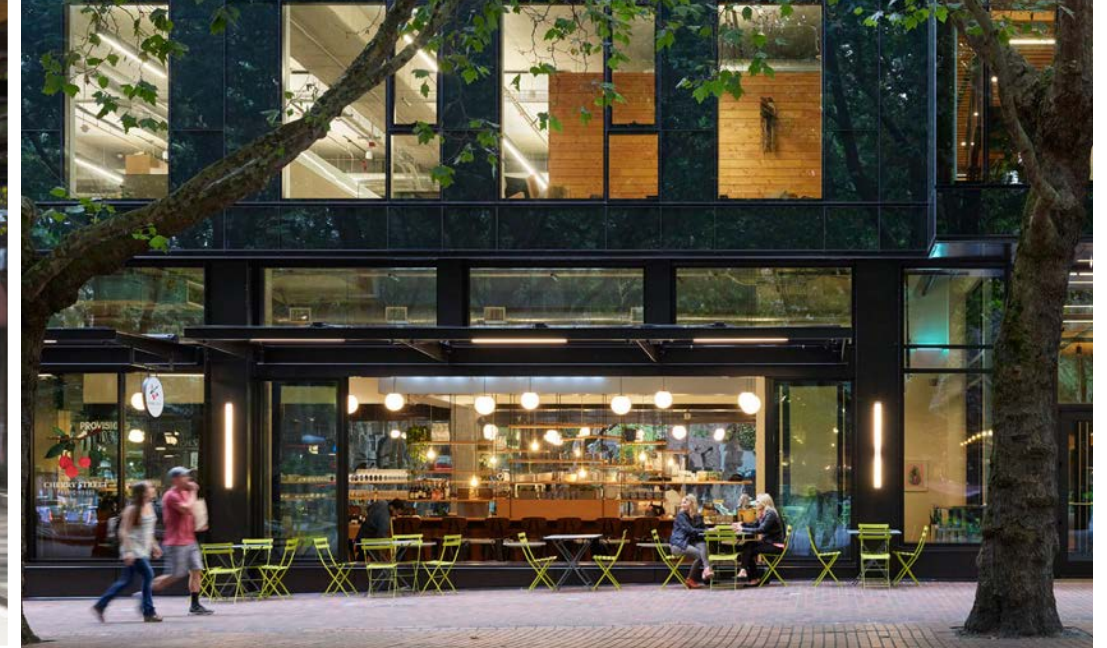
Moveable walls and partitions can activate the theatrical quality of the building facade
