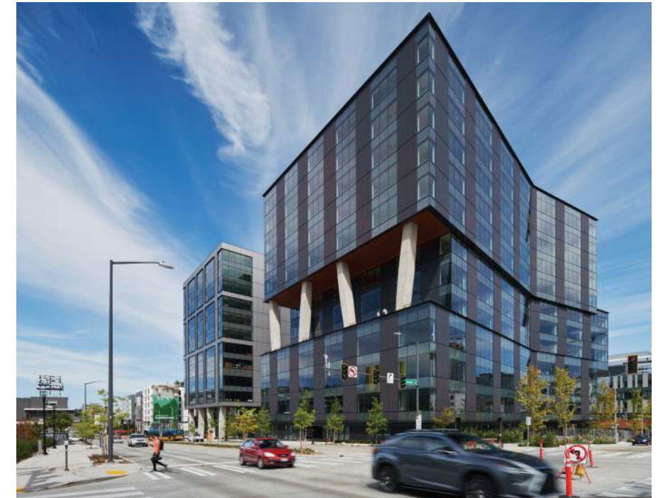
333 Dexter, Seattle, design by Miller Hull (Completed 2021)
