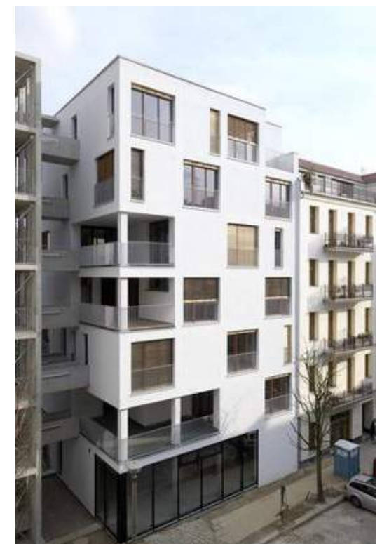
E3 building - Kaden Klingbeil
