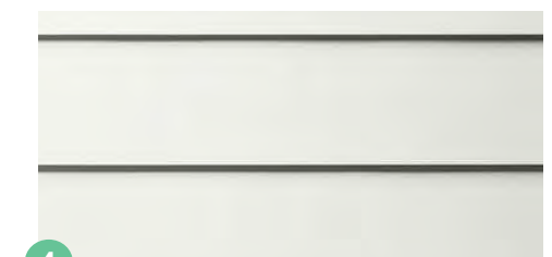
4 SMOOTH CEMENT LAP SIDING AT LOWER FLOORS AND STAIR TOWERS
