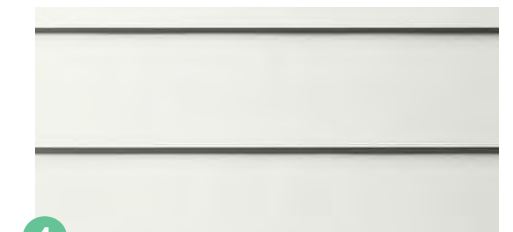
4 SMOOTH CEMENT LAP SIDING AT LOWER FLOORS AND STAIR TOWERS
