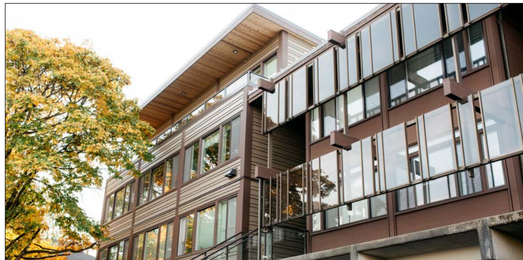
MOD (THEODORA) APARTMENTS (LANDMARK, GRANT, COPELAND, CHERVENAK & ASSOC.)
