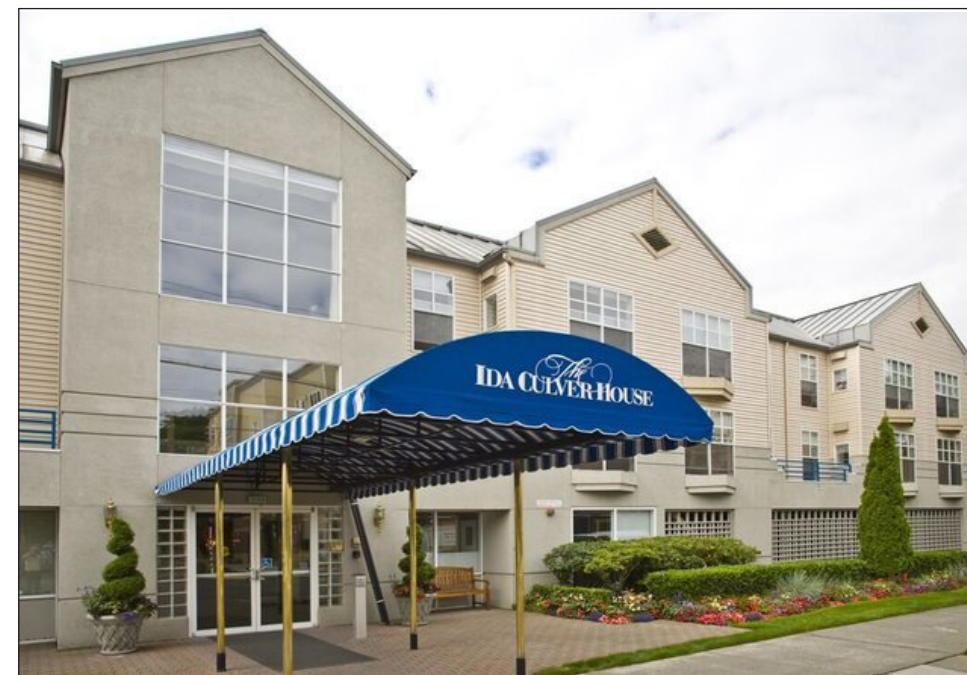
IDA CULVER HOUSE RAVENNA, 1988 ADDITION
