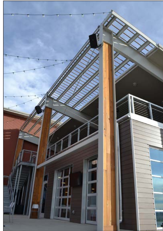
EXPOSED BEAMS & COLUMNS
