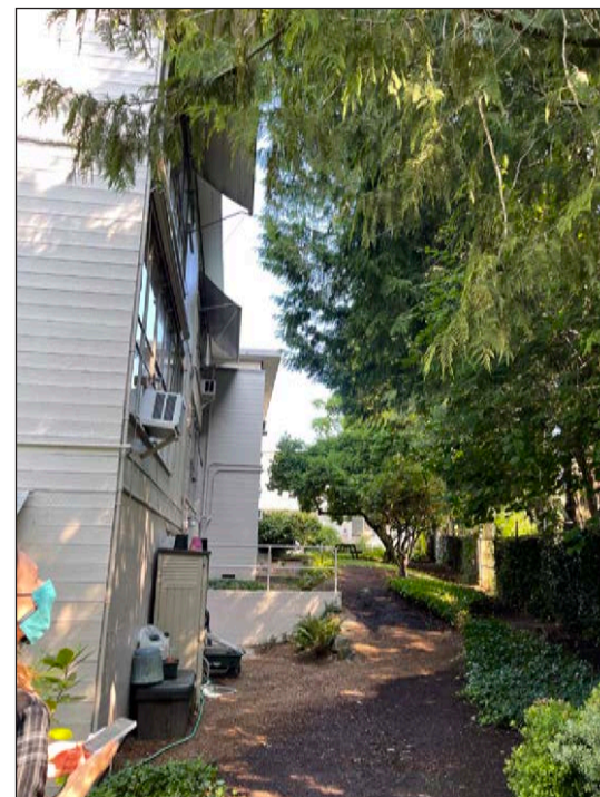
THREE-STORY PORTION OF EXISTING STRUCTURE AT SOUTH END OF SITE
