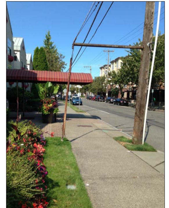
UTILITY POLE WITH GUY WIRE AT N 65TH ST RIGHT-OF-WAY
