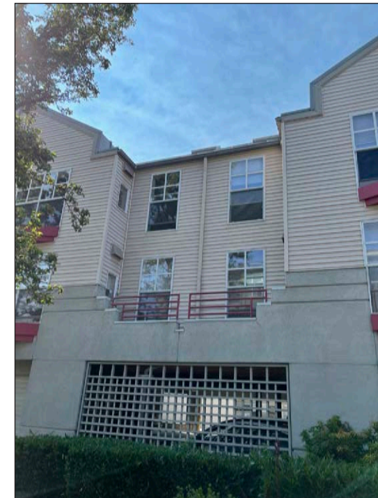
SCREENED PARKING ALONG STREET- LEVEL FACADE ON N 65TH ST
