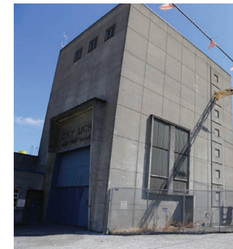
6 Seattle City Light Broad Street Substation (50') 565 Harrison St.
