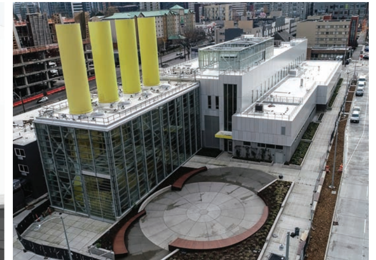
14 SR-99 North Portal Tunnel Operations Building (50')
