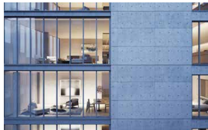
Exposed Concrete Shear Wall
