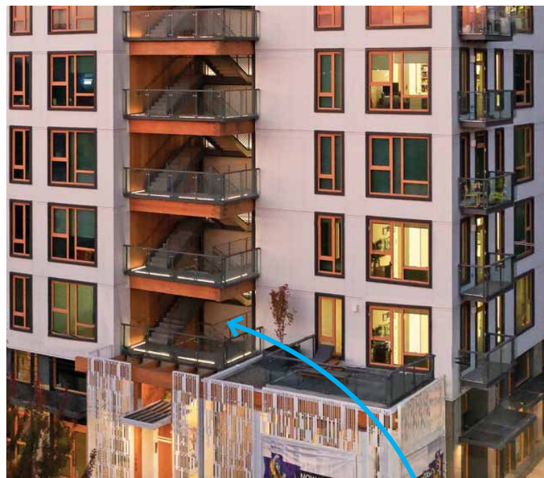
SOLIS APARTMENTS — WEBER THOMPSON
