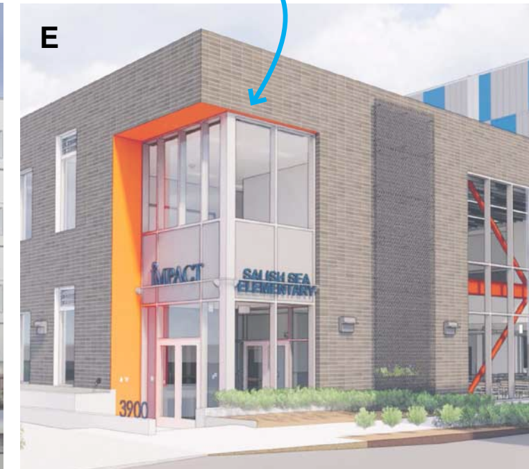
E SALISH ELEMENTARY SCHOOL (UNDER CONSTRUCTION) Solid block with punched openings
