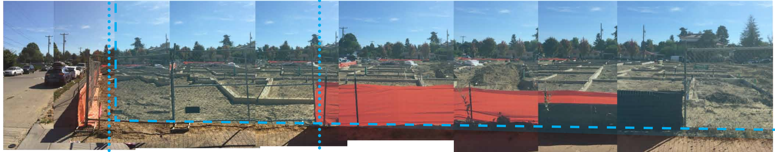
4031 S WILLOW ST 6905 - 6931 42ND AVE S TOWNHOUSE/ROWHOUSE DEVELOPMENT (UNDER CONSTRUCTION)
