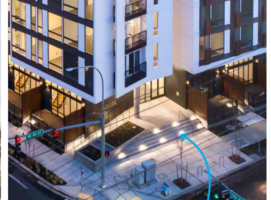
STATION HOUSE — WEINSTEIN A+U
