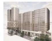
14 & 15 Residential + Office 4522 Roosevelt Way NE 22 stories & 16 stories
