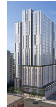
6 Core Tower 4515 + 4525 Brooklyn Ave NE 24 stories
