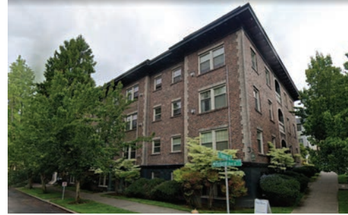
1052 E THOMAS ST [APARTMENTS] Four-story multi-family. Strong contrasting color building base. Brick upper facade volume that contrasts base. Building corners accented with stone. Large bay-windows with accent trim. Lush planting buffer between building and sidewalk.
