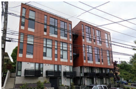
1202 E THOMAS ST [APARTMENTS] Six story multi-family. Strong double-height base. Upper facade contrasts base and groups windows vertically to form tall bay-windows with accent trim. Main entrance tucked between volumes.
