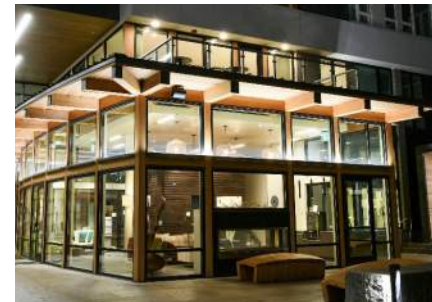
3 LED MULLION MOUNTED LINEAR UPLIGHT FOR ILLUMINATION AT FEATURE SOFFIT
