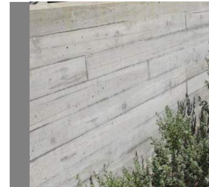
BOARD FORM CONCRETE SITE WALLS
