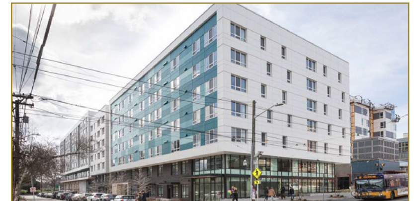
Station House TOD | Seattle, WA
