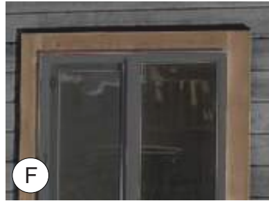
F TIGHT KNOT CEDAR (TONGUE & GROOVE) STAIN: WOODSCAPE THICKNESS: 1" SIZE: 4" X 144"
