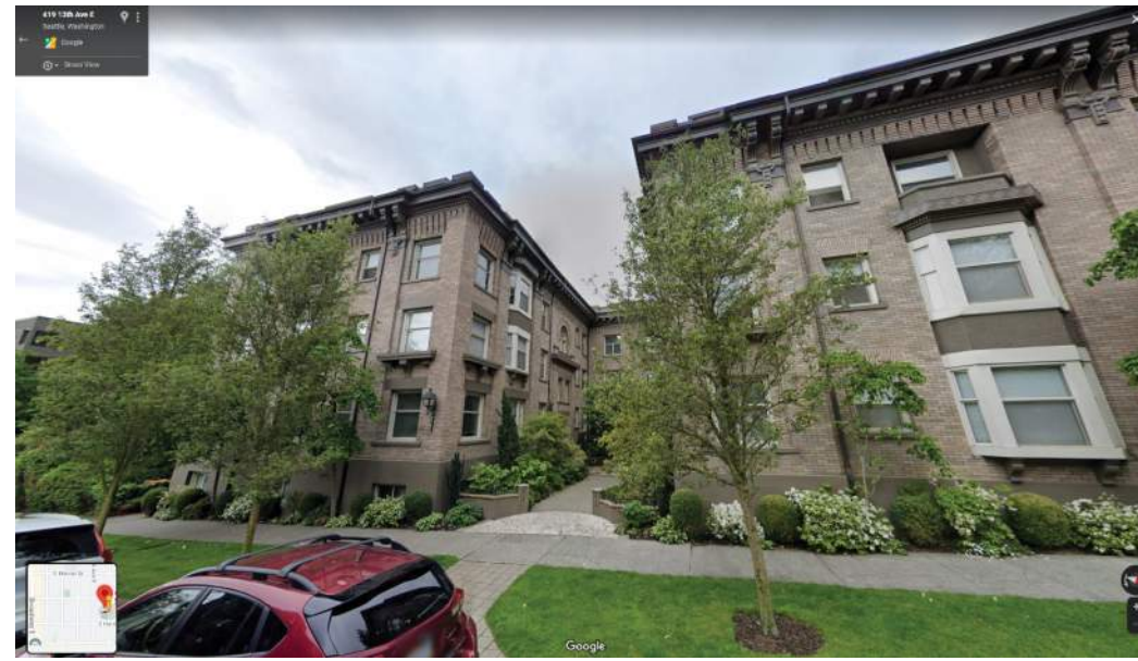
Hampton Court - different material treatment at "garden" units versus upper mass to shorten build appearance, recessed courtyard entry is easy to find, deep punched windows provide relief on bold & symmetrical massing
