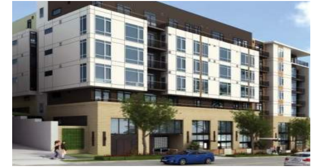
Avalon Way Apartments - pop-out articulation leads to lack of spatial legibility, hard to find entry at street-level
