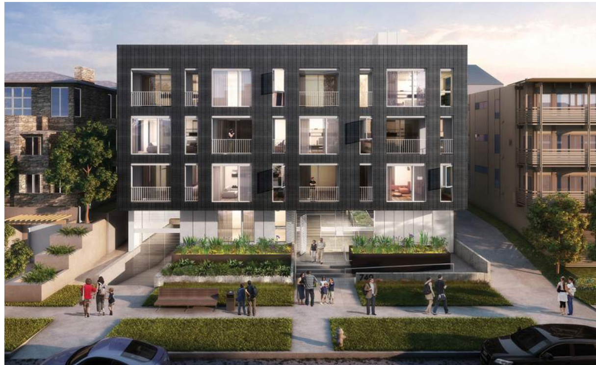
Harvard Too (under construction)
