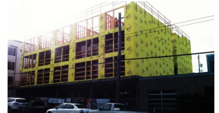
⑪ 1315 East Jefferson Apartments - In-construction.
