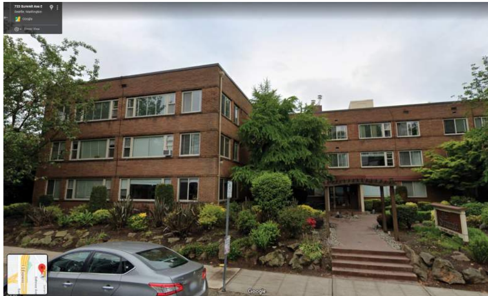
The Summit - deep courtyard reduces perceived bulk/density, landscaping draws sidewalk activity in, toward entry. strips of varied windows create rhythm within a field of homogenous material
