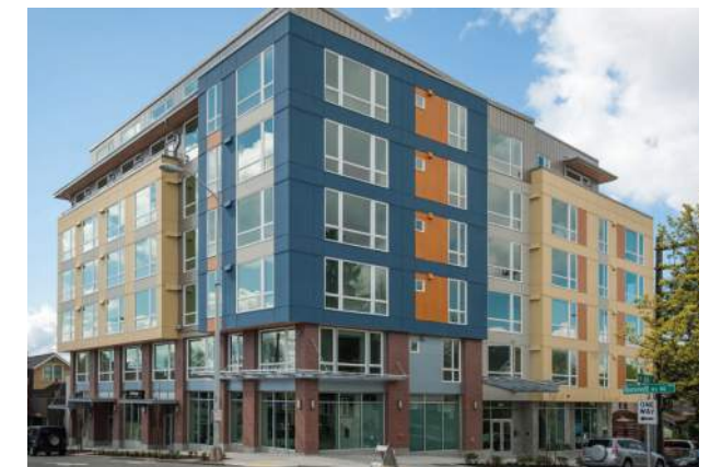
The Kavela Apartments - garish colors and blocky composition make for a busy-looking and placeless building
