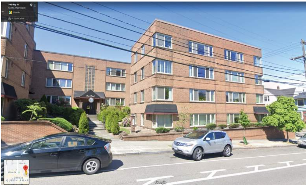
Roy Street Apartments - awnings at street level units reduce scale for a more residential look. height and mass do not impose on adjacent single family houses. punched windows provide depth to flat facade
