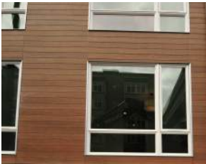
Example of Nichiha panel with vinyl flanged VPI window.
