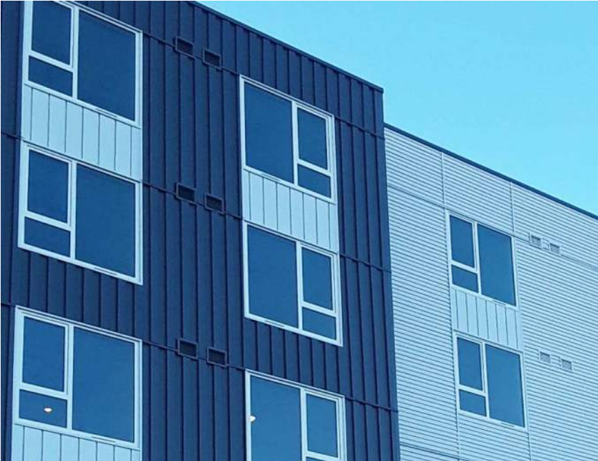
Color Matched Xvent Installation in Metal Siding
