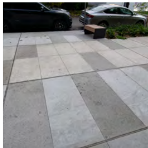
Paving at Plaza
