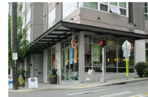
Canopy defining entry & corner
