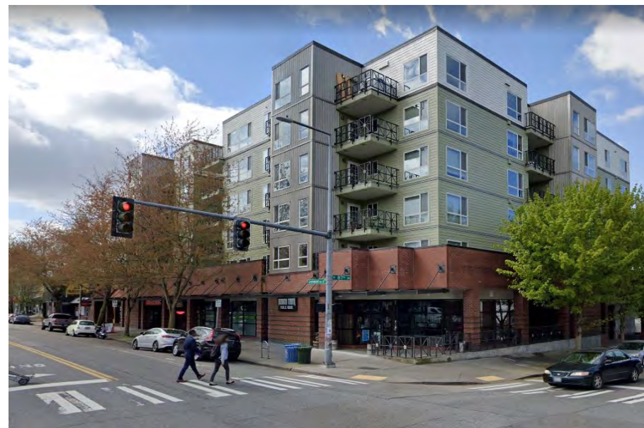
Towers on Greenwood - 8551 Greenwood Avenue N (Google)
