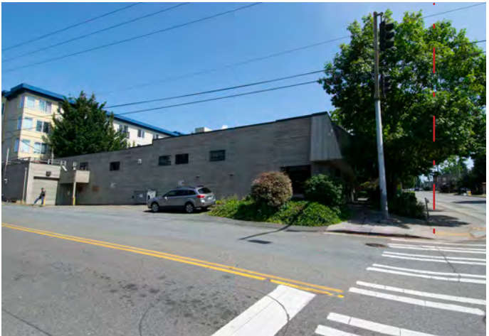
2. Looking northeast from N 85th Street
