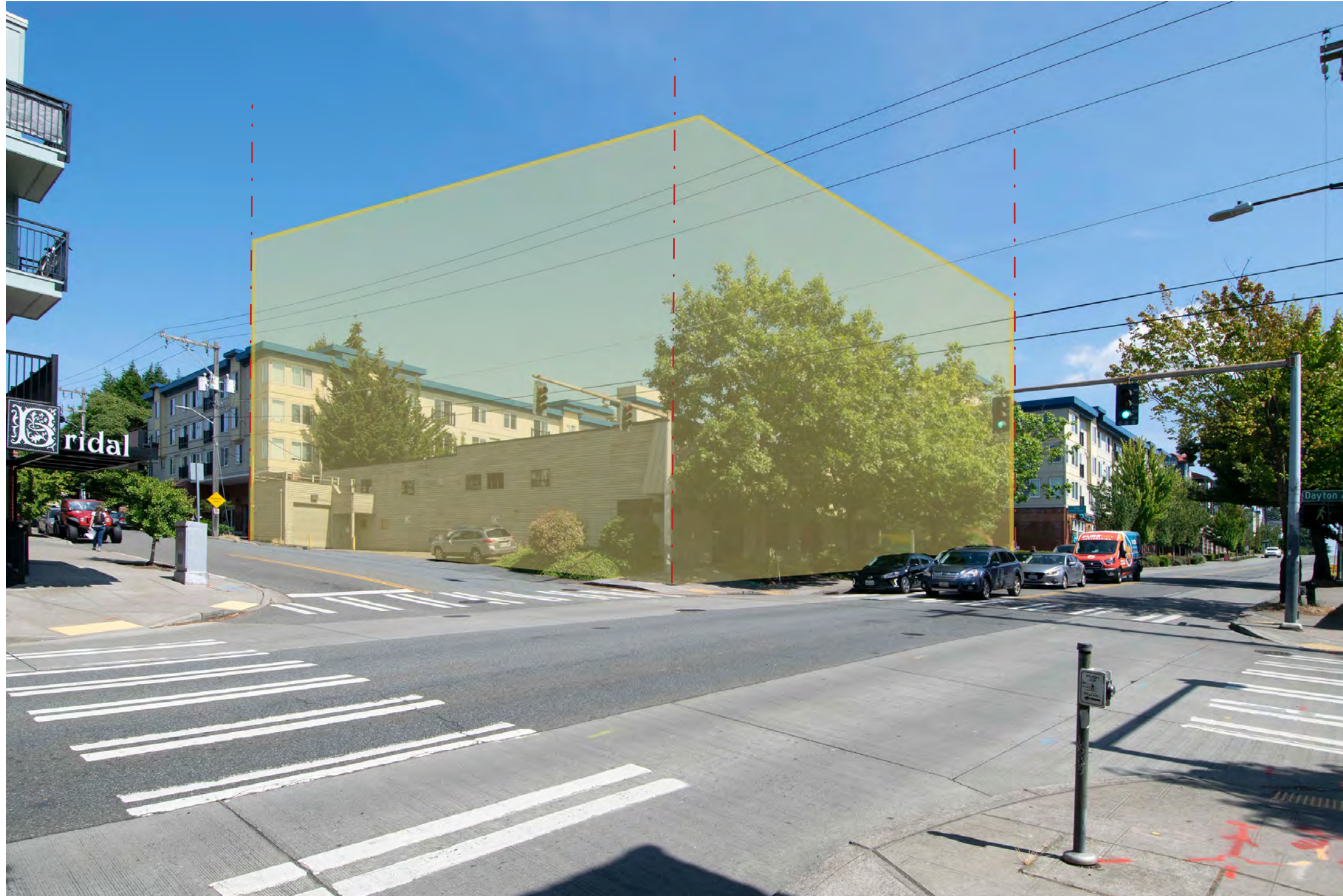
Looking northeast from N 85th Street
