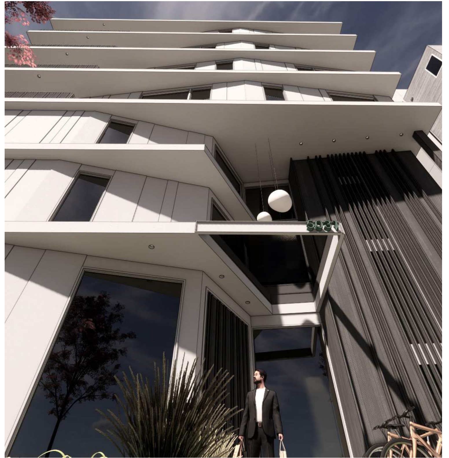
EAST FAÇADE VIEWED FROM BELOW
