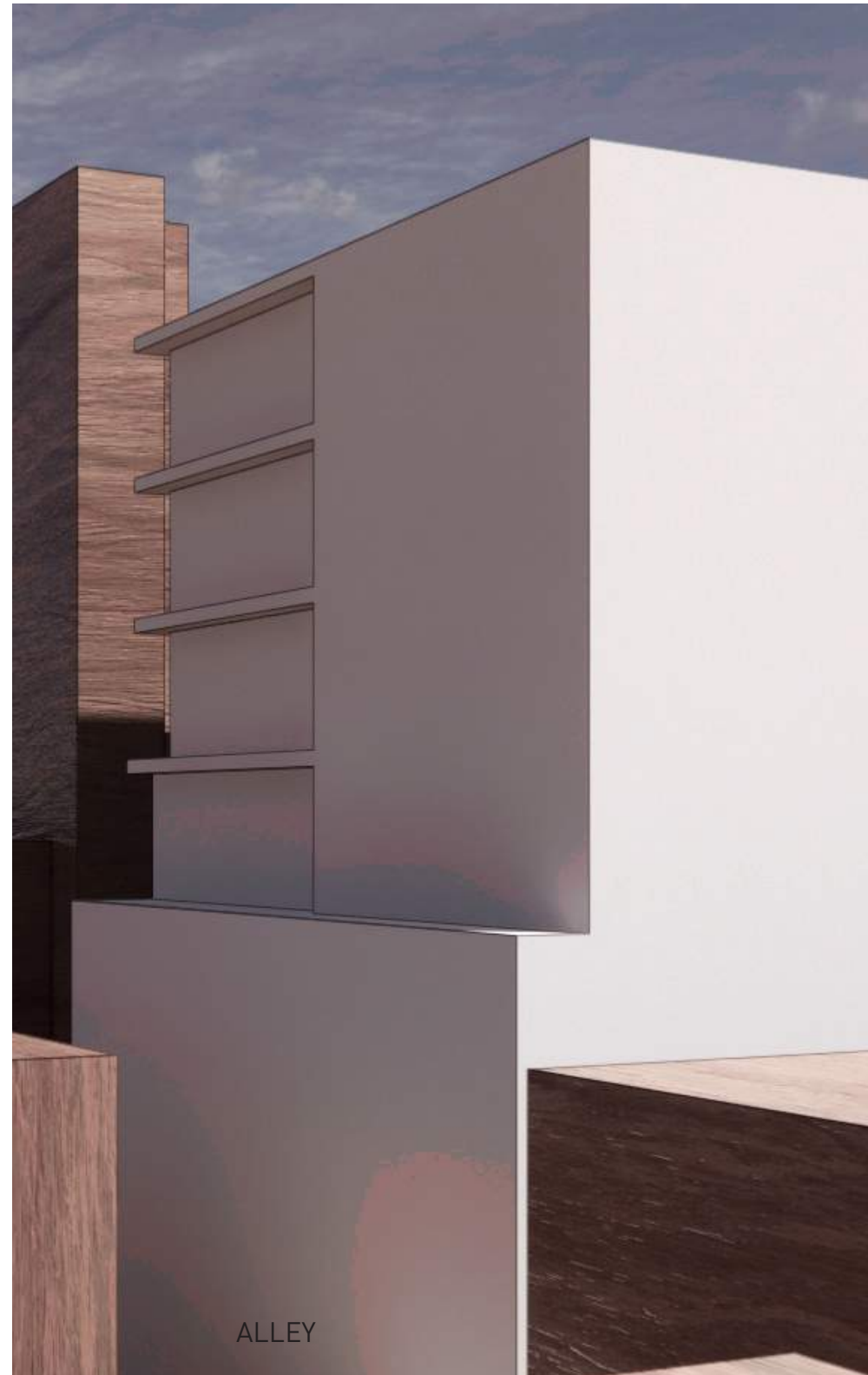
SOUTHWEST (ALLEY) VIEW
