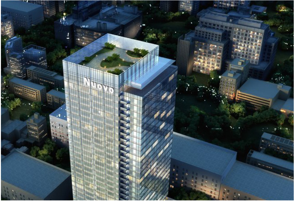
FACADE TREATMENT AT ROOFTOP
