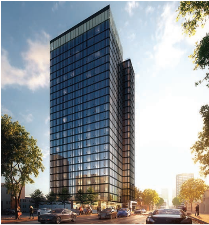
2 - THE M 4700 BROOKLYN AVE NE Residential | 240ft | 24-story #3028621-LU
