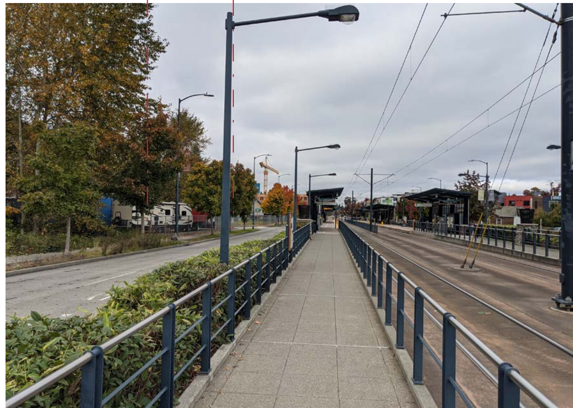
1. Looking north on light rail platform
