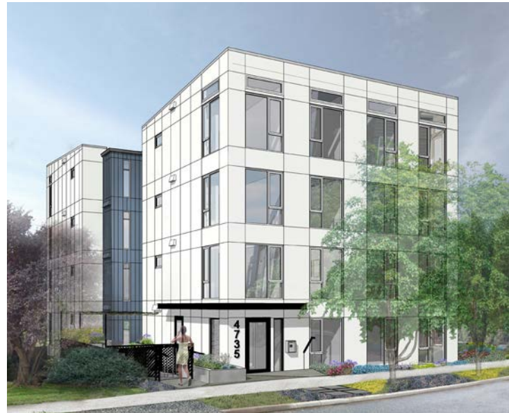
4735 32nd Ave S (Under Construction)
