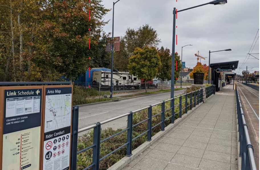
4. Looking northwest from Martin Luther King Jr Way S (Link Light Rail Platform)
