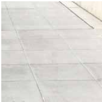
2'x2' city standard ROW paving (No Shiners)
