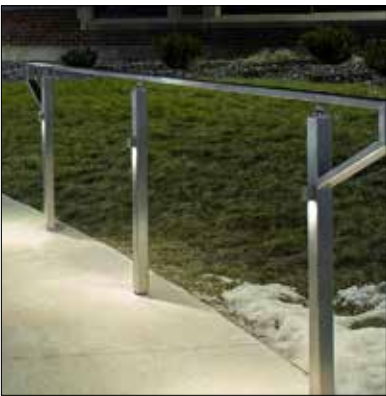
3 Handrail Lighting Lights mounted to handrail stanchions illuminate terrace perimeters.
