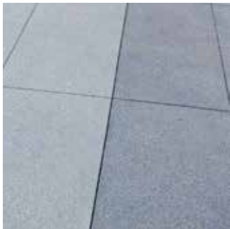
Specialty concrete paving w/ sawcut joints (w/ integral color)
