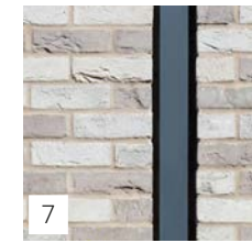
7 Recessed Metal Downspout at Brick, Prefinished Black
