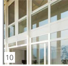
10 Prefinished Flat Metal Infill Panel, Aep Span 'Regal White', W/ Aluminum Storefront Windows, Arcadia Finish to Match Infill
