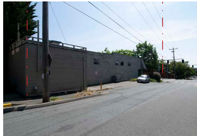
1. Looking southeast from Dayton Avenue N
