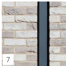
7 Recessed Metal Downspout at Brick, Prefinished Black
