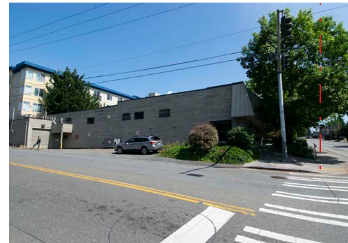
2. Looking northeast from N 85th Street
