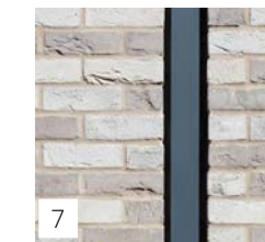
7 Recessed Metal Downspout at Brick, Prefinished Black
