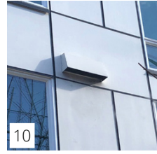
10 Exhaust Vent Shroud at Fiber Cement, Paint to Match Field
