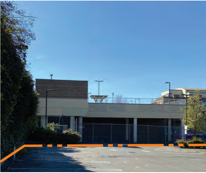
5 LOOKING SW THROUGH SITE
