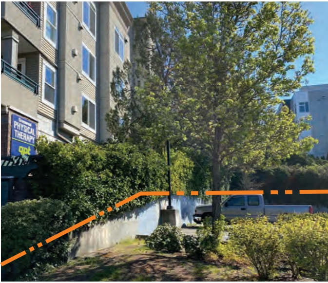
4 LOOKING S THROUGH SITE
