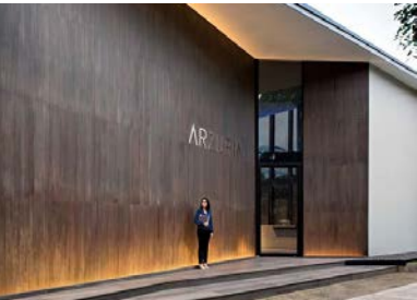
peeling the mass back at the residential lobby clearly identifies the entry and provides weather protection overhead (PL2.C2, PL2.D1)
