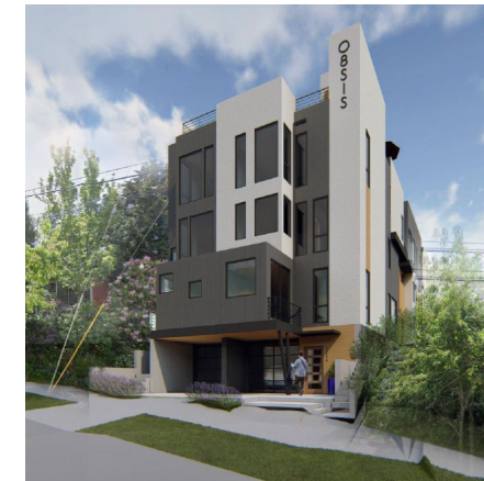
2. 1317 N 44th St 3 Story, 8 Units, 3 spaces Under Construction
