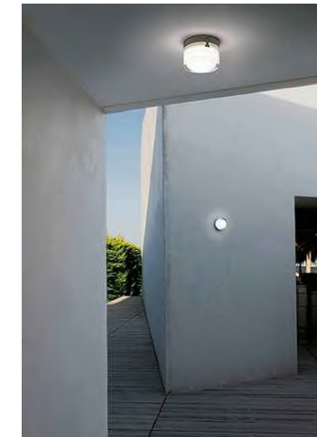
① surface mount wall or ceiling lights at entries and overhangs
