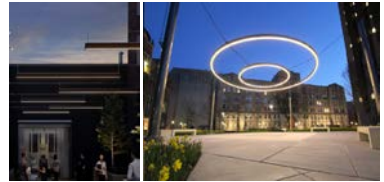
SH1 & SC1, SC2 SPECIALTY CATENARY FIXTURES MOUNTED UNDERNEATH THE BUILDING CONNECTORS
