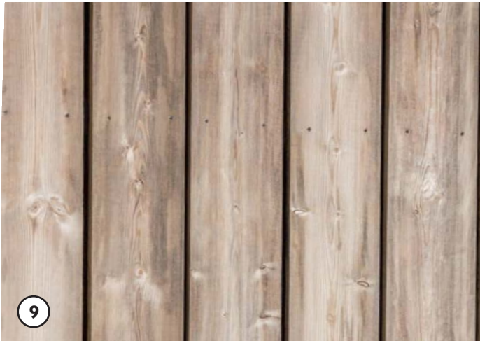
9 THERMALLY MODIFIED WOOD CLADDING / SCREENING 1x6 SHIPLAP (KEBONY OR SIMILAR MFR)
