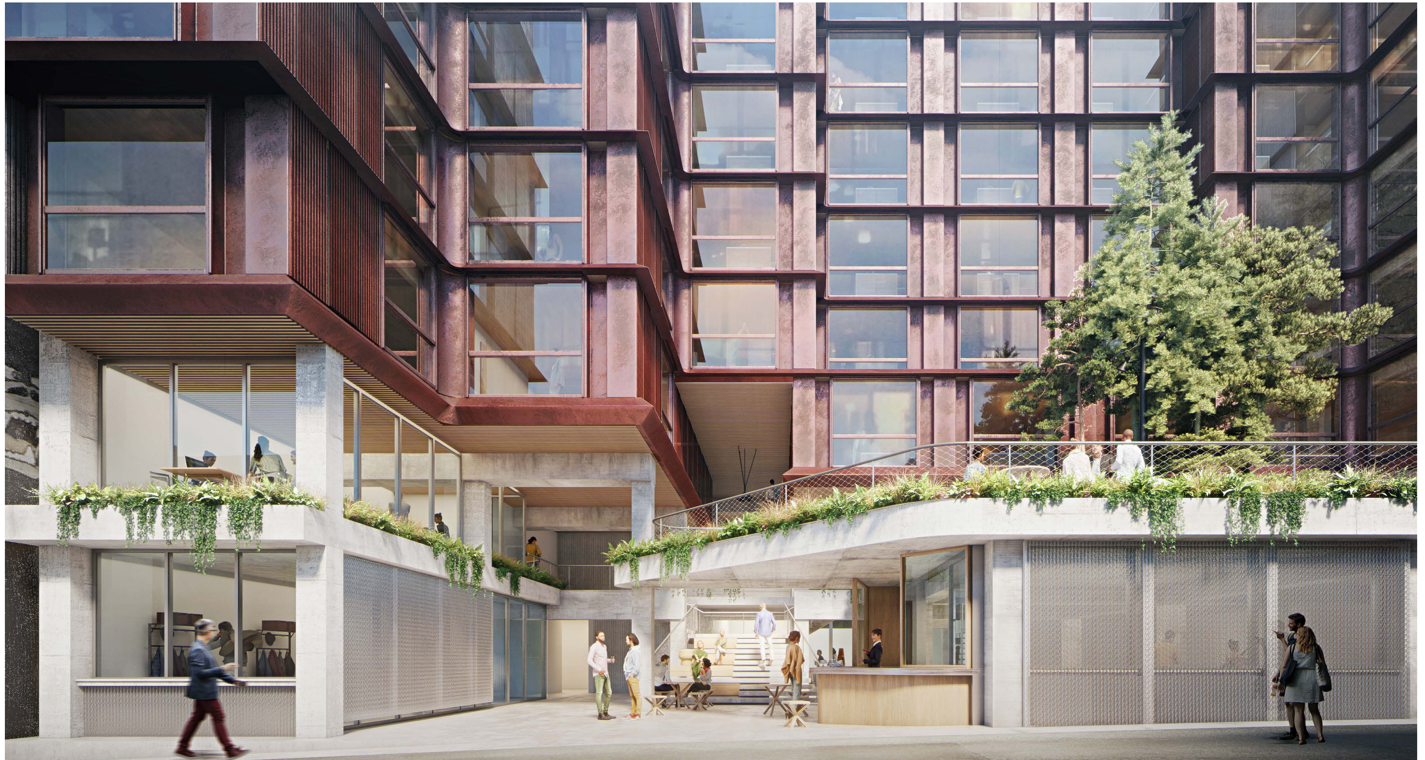
View from the Alley looking into the laneway and the new central stair
