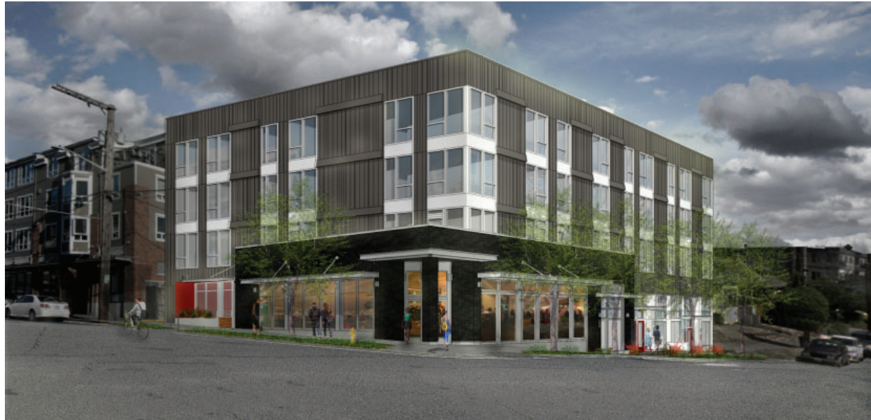
800 5th Avenue N (Under Construction)
