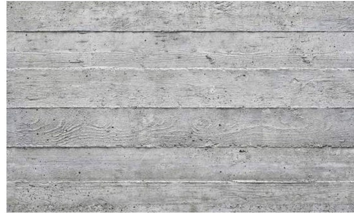
Bio-retention planter edges along sidewalk are cast in place board-formed concrete
