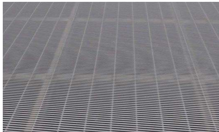
Bridge elements at entries on street level are metal grating that will develop a patina over time
