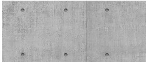
⑥ CAST-IN-PLACE CONCRETE SMOOTH FINISH
