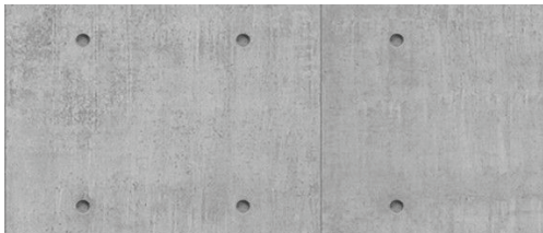
⑦ CAST-IN-PLACE CONCRETE SMOOTH FINISH, SNAP-TIE PATTERN
