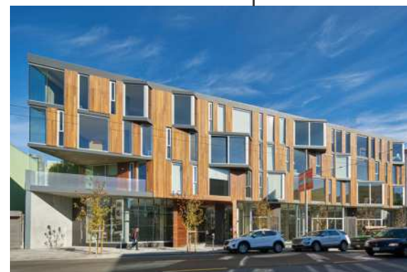
Facade and window opening modulation
