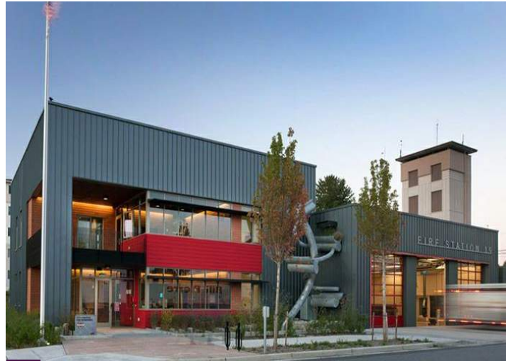
7 Lake City Fire Station
