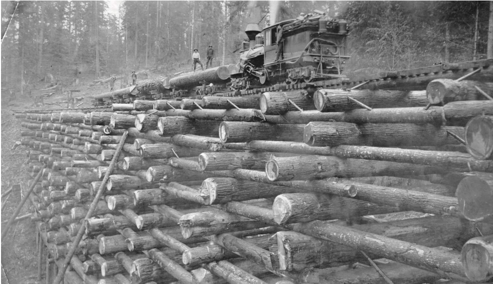
Timber Crib Trestle Bridge along Northern Pacific Railroad
