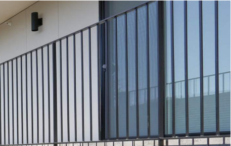
6 GUARDS // POWDER COATED STEEL // CHARCOAL 1 1/2" X 1/2" STEEL FLATBAR VERTICALS, 4" O.C. SPACING
