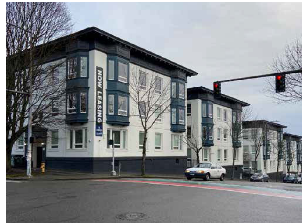
④ VICTORIAN / EDWARDIAN APARTMENT BUILDINGS
