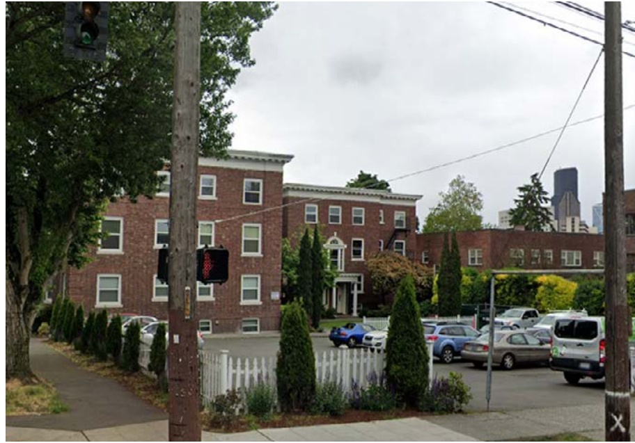
Existing Helen V apartment building, looking South from the corner of East Union St. and 14th Ave.
