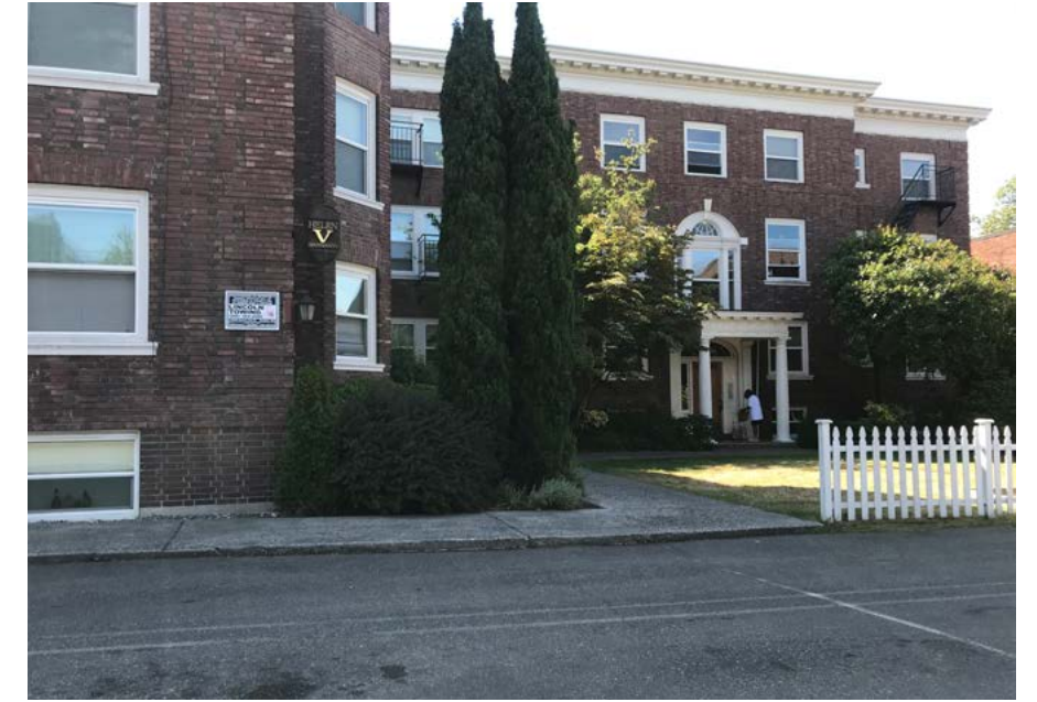
Existing Helen V apartment building, as viewed from the parking lot in front - to become the shared courtyard once the proposed building is constructed.
