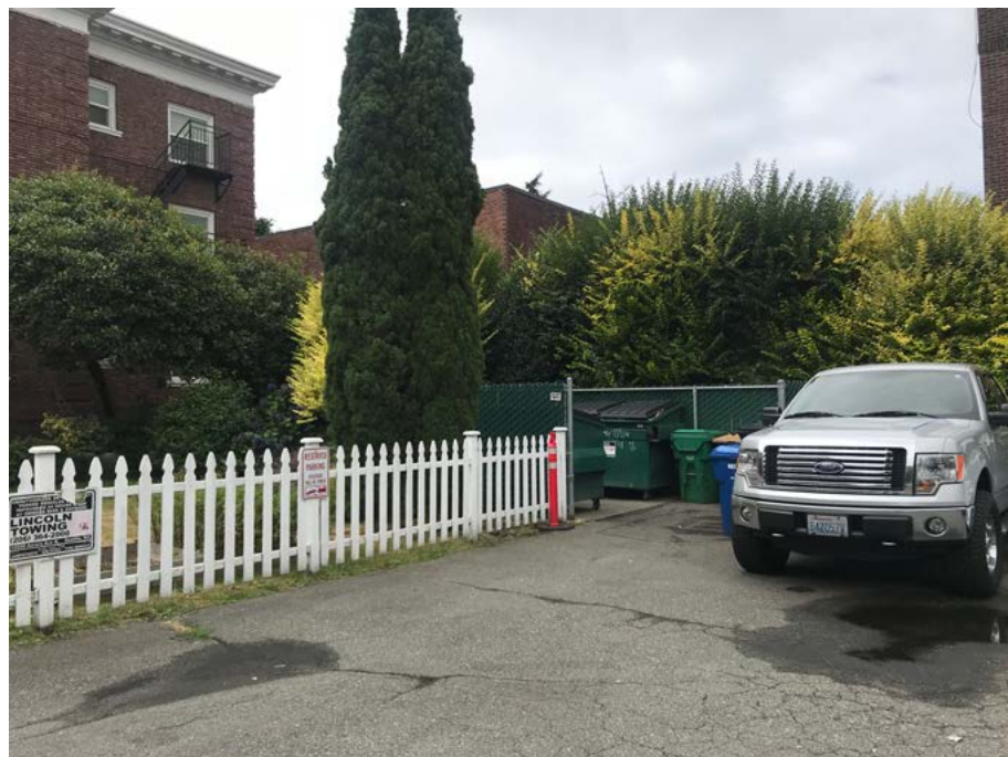
Access to the trash enclosure in front of Helen V, at the South-West corner of the existing parking lot.
