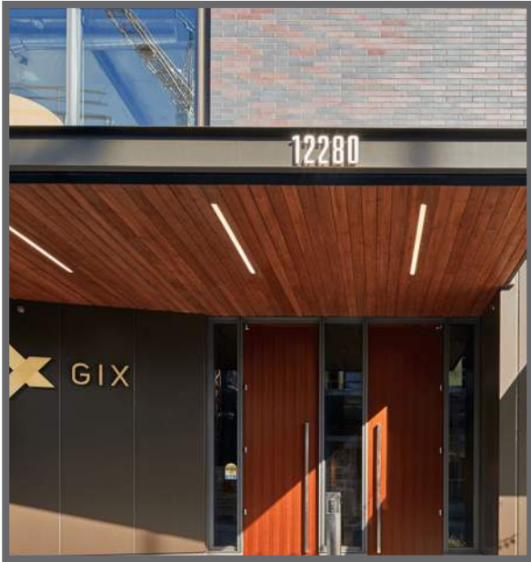
5 Linear Canopy Lights- Recessed linear lights at wood soffit canopies. Finelite- HP-4 WL R
