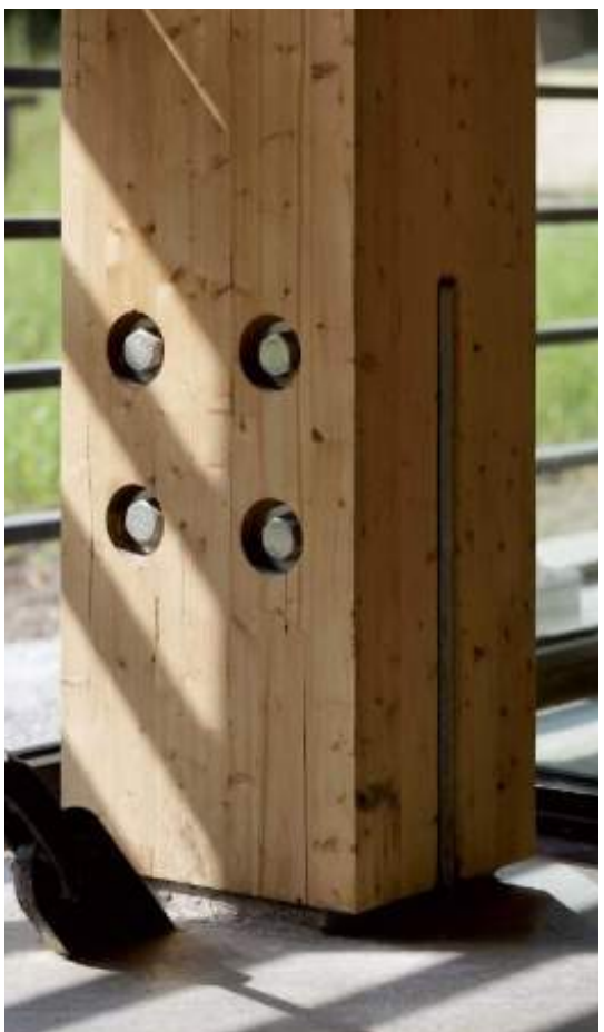
1 POST BASE ATTACHMENT DETAIL
